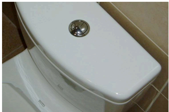
Fig. 1: Residential dual flush button design
